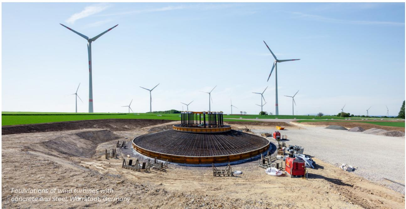
*Foundations of wind turbines with concrete and steel, Wörstadt, Germany*
