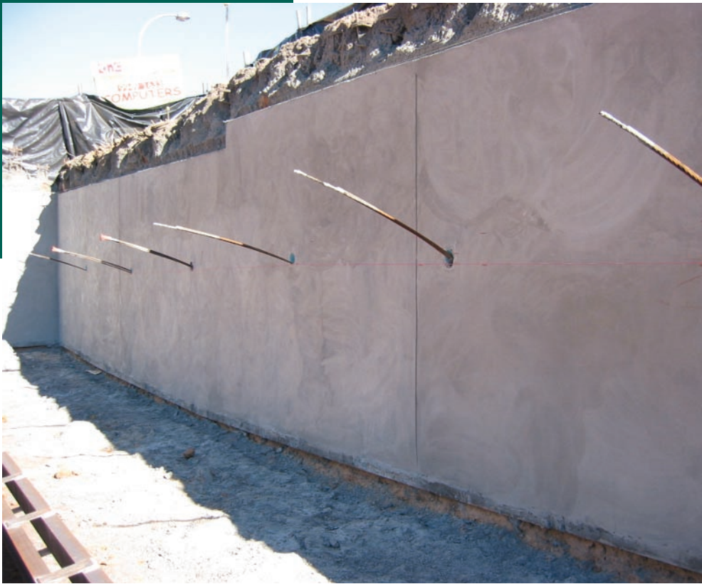
ABOVE: PREPARED RETAINING WALL BEING SPRAYED LEURA BY PASS. LEFT: SHOTCRETE WOOD FLOAT SPONGE FINISH.
