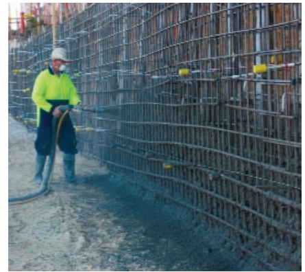
ABOVE: PREPARED RETAINING WALL BEING SPRAYED LEURA BY PASS. LEFT: SHOTCRETE WOOD FLOAT SPONGE FINISH.
